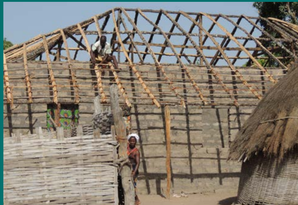
Montagem de telhado com barrotes de Borassus aethiopum | Roof assembly with joists from Borassus aethiopum , Guiné-Bissau. Luís Catarino, 2013
